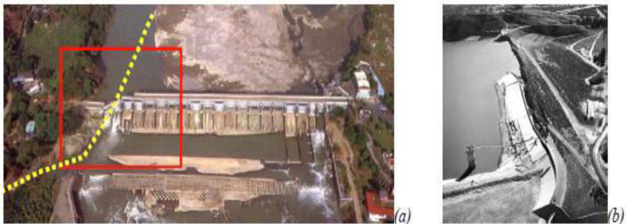
Figure 3. Earthquake-related geohazards and failure of dams: (a) collapse of the concrete Shih-Kan Dam during the 1999 Chi-Chi earthquake in Taiwan due to active fault rupture, (b) severe damage to the Lower Van Norman Dam during the 1971 San Fernando earthquake in USA.
